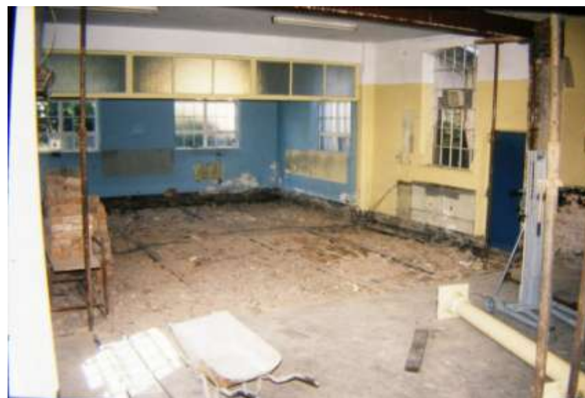
Renovation underway in the rear hall
