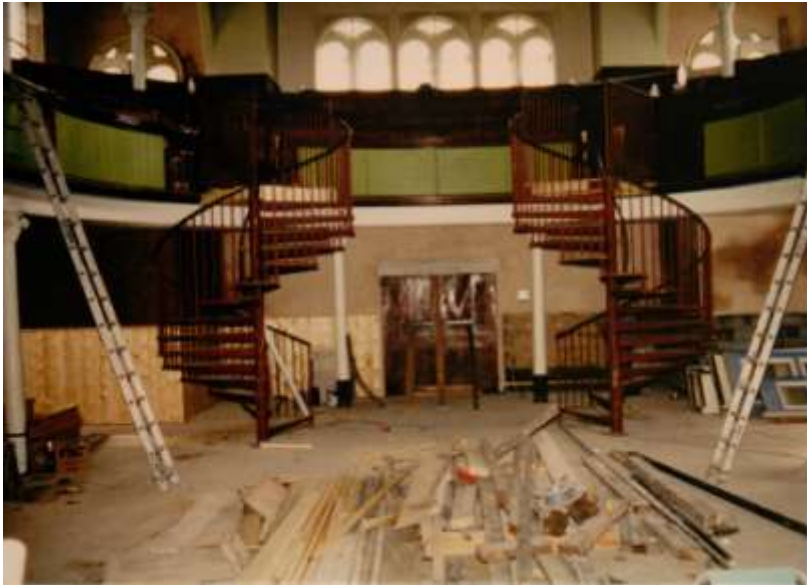
New spiral stairs to gallery installed
