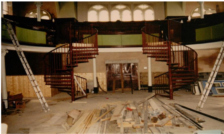
New spiral stairs to gallery installed.
